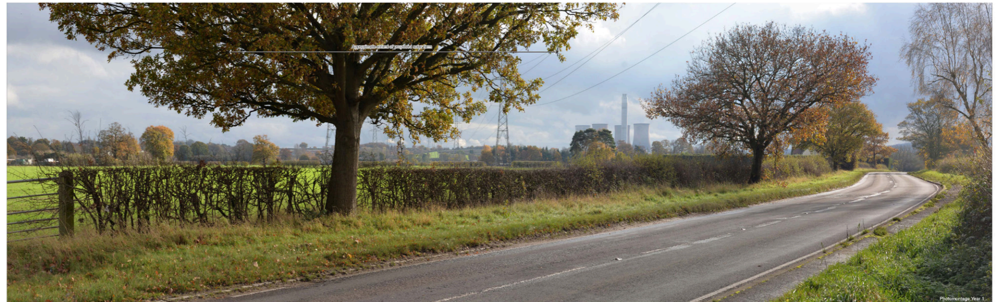
Figure 6B VP7- View from junction of Colton Road and Staffordshire Way recreational route with solar farm and soft screening superimposed, year 1.
