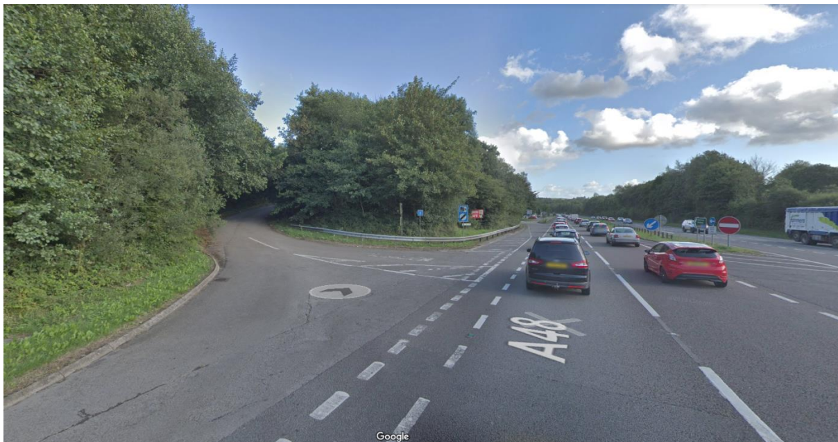
Photo 4: Exit from A48 southbound onto unclassified road to Area 3
