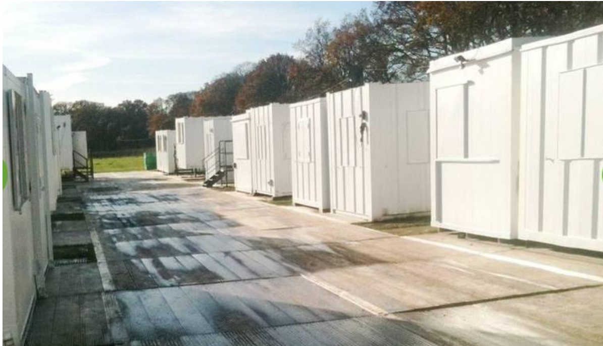
Figure 7 – Aluminium trackway used to provide hardstanding within a construction compound
