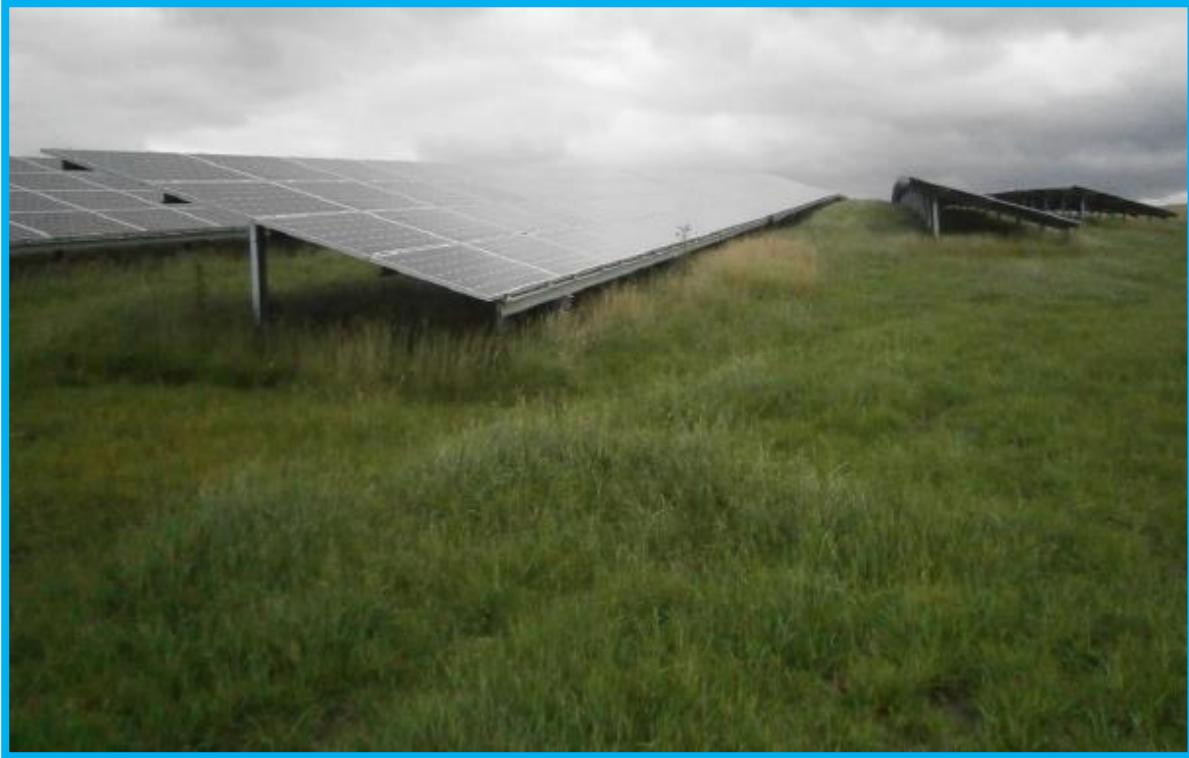
Fig 12 Solar arrays on 1 in 8 slope showing flourishing vegetation (Merthyr Tydfil).
