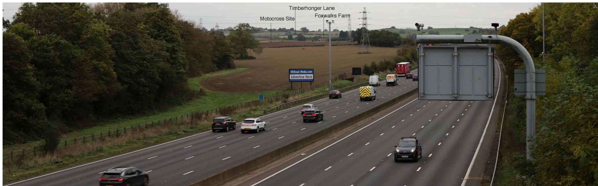
VP12 - View from the road bridge west of Upton Warren looking north.
